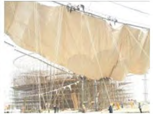
On site assmebling of the membrane.
