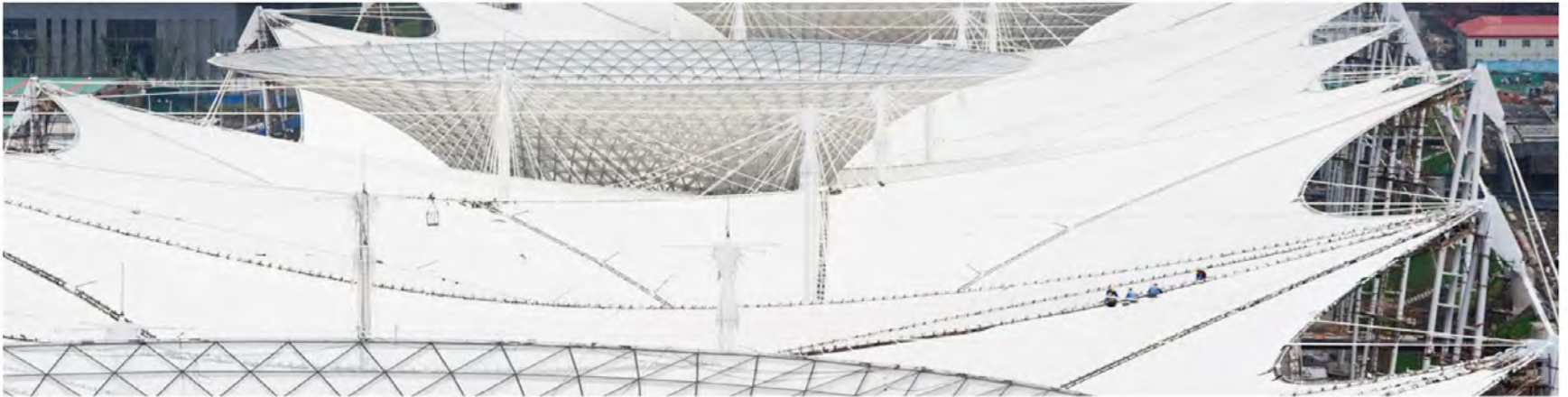
On site assmebling of the membrane.
