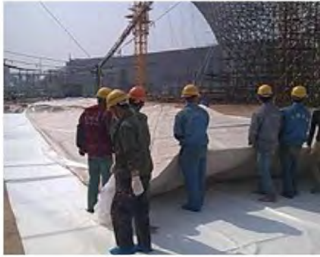
On site assmebling of the membrane.
