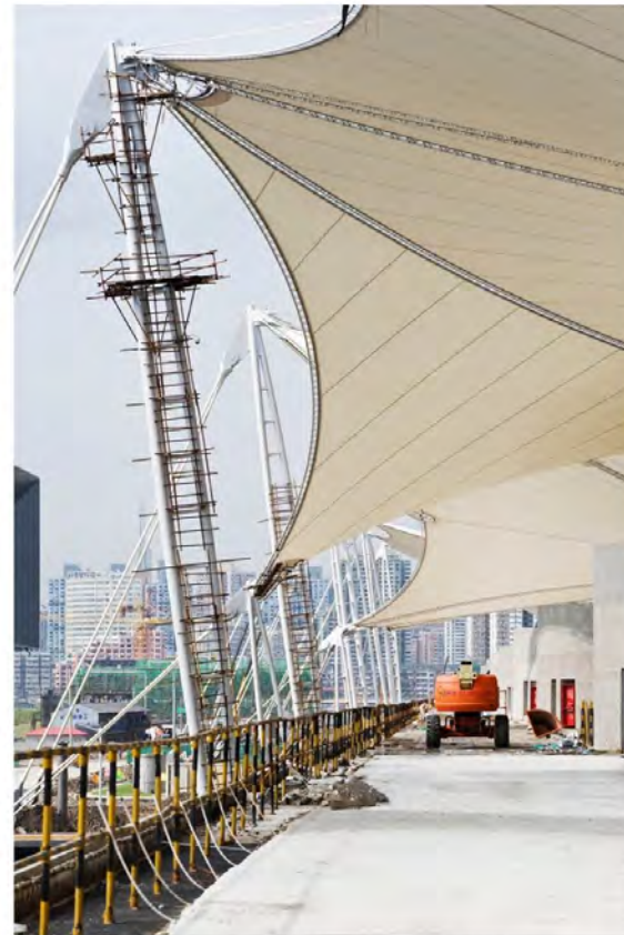
Assemble the mast with the Membrane
