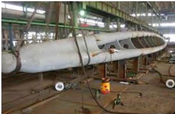
Assembling the mast
