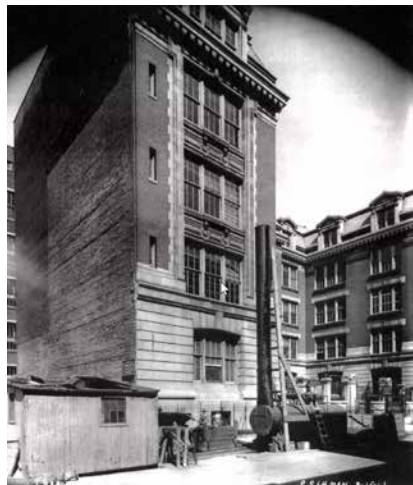
081_PS64_104 Finishing touches on a new school, 1906
