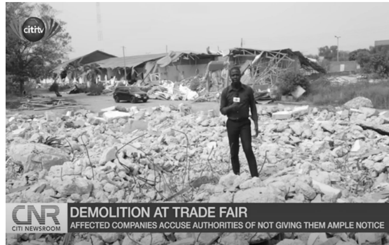
009_ARLL_108 Demolition of over 2,100 small businesses, 10:00 pm on February 16th, 2020
