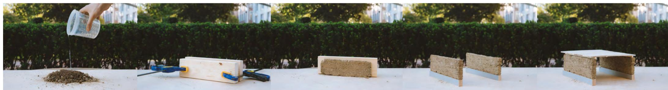
Rammed Earth construction is unique in its circular life process, which means that the prefabricated panels are not mixed with any additional materials, so the soil can be reused over and over again, whether material for a new building, or back into the landscape. Studies have shown that stabilized rammed earth with cement does not produce large structural advantages, while at the same time breaking the circular life process of rammed earth.
