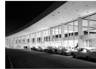
SOM came up with an elegant, two-level, crescent-shaped building providing 250,000 sqft of floor space. The facade, which spanned 691, was constructed entirely of glass panels and aluminum frames. A double-height check-in hall in the center of the building was flanked by baggage claim areas.
