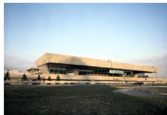
GMW designed a functional three-level structure of reinforced concrete and tinted glass, in the style of Brutalism, which was popular in Europe at the time. The terminal featured a flat overhanging roof and inward sloping walls. In the initial design, the 300,000 sqft terminal featured a pier which could accommodate six BOAC VC-10s.
