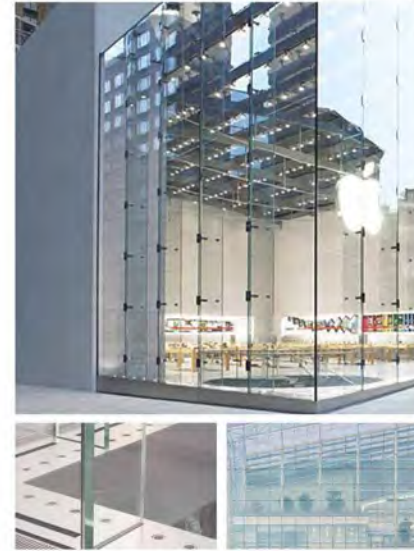
1. Glass Transparent New Interior Facade
