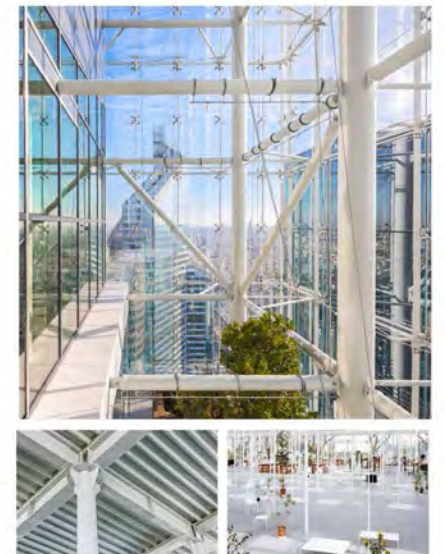
4. Steel White Main Structure
