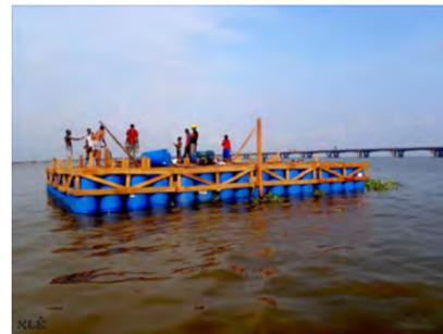
Figure 2: The project uses barrels to achieve the purpose of floating, from NLE official website
