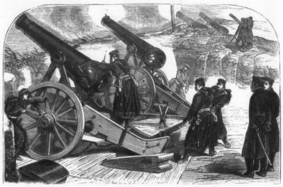
STEGE OF PARIS.—MANNER IN WHICH THE PRUSSIAN SIEGE-GUNS ARE MOUNTED, BY ELEVATING ABOVE THE CARRIAGES, SO AS TO AVOID LARGE EMBRASURES IN THE BREASTWORK.
