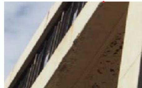
Spalling concrete at the edges of the building
