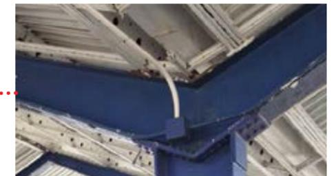
Corrosion on the steel frames
