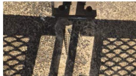
Spall on the concrete coping
