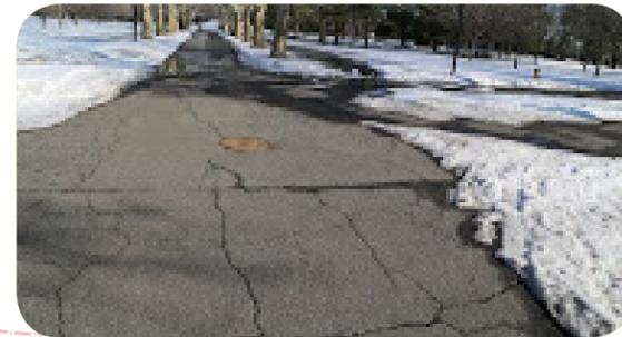
Cracked and uneven pavement
