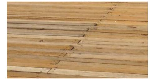
Uneven surface on the timber deck
