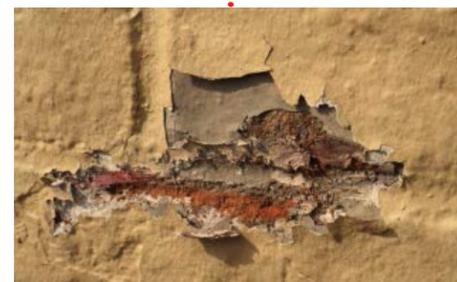
Spalling bricks covered by paint layers
