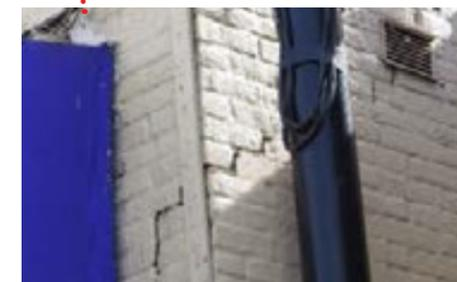
Cracks at the corner of right staircase
