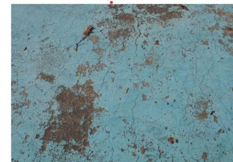
Cracks at concrete pool
