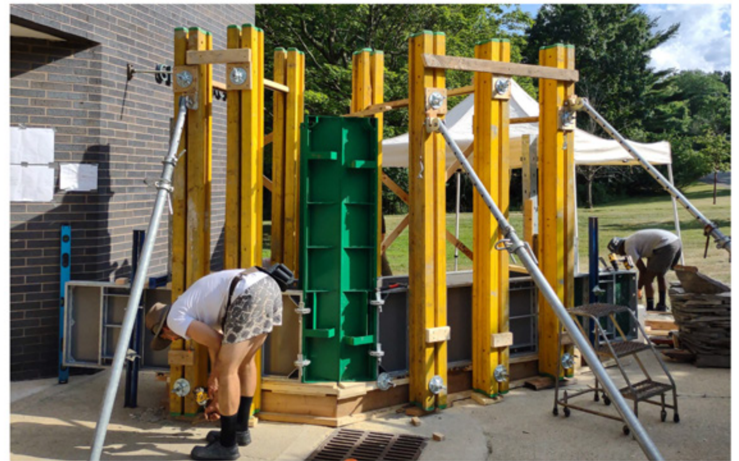
Formwork assembly
