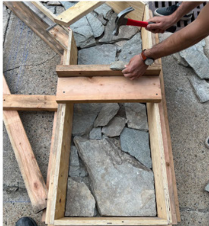
Footing masonry construction
