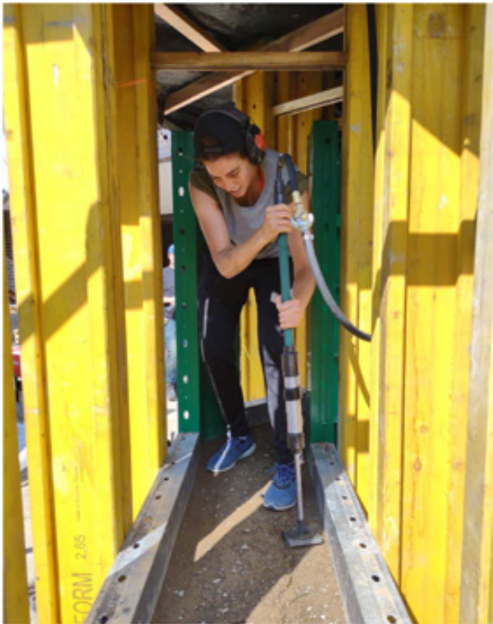
Steps for ramming process
