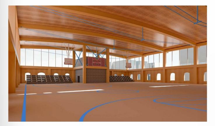
Long span glulam with steel tie rod at gym
