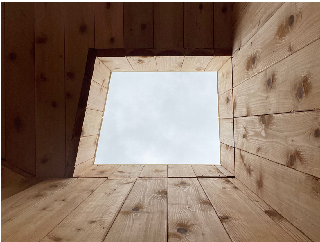
Construction photos, October 2021
