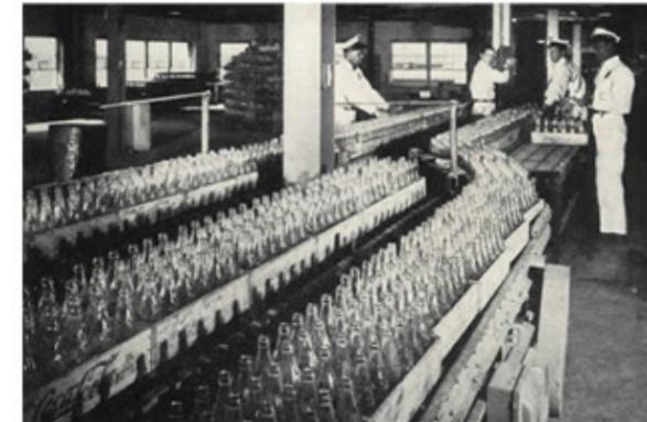
The Coca Cola bottling plant was originally built in 1950, when there were three buildings on the site, for bottling, drive through, and storage/advertising and repair. The prototype was designed by the architects Stone and Pitts, to provide maximum efficiency, which combined the skill of workers and the efficient of machines to bottle 1,280 bottles per minute.
