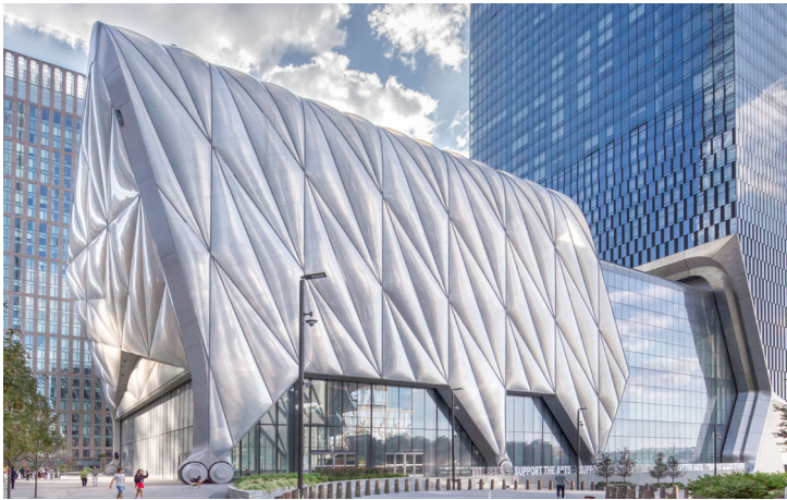
The Shed's façade from the north across Hudson Yards Public Square. (Photo: Brett Beyrer.)
