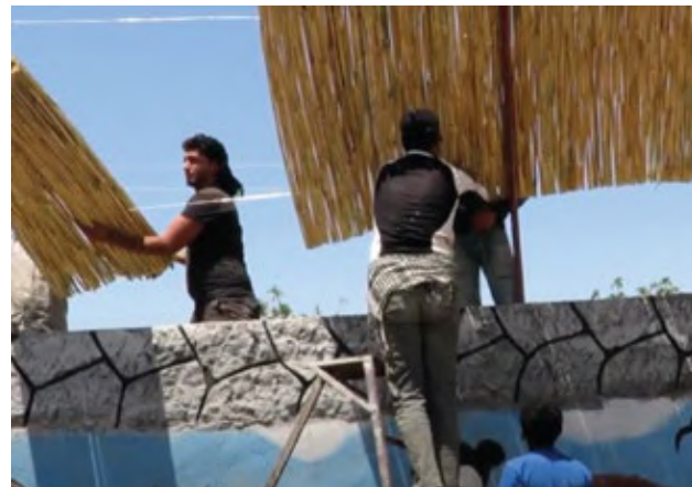
Men Constructing Shade Awning using Al-Kassab Reed. 18
