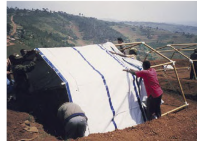
Paper Emergency Tube Shelters in Byumba Refugee Camp, Rwanda. 22
