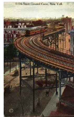
Fig 1 110th Street Elevated Curve, New York
