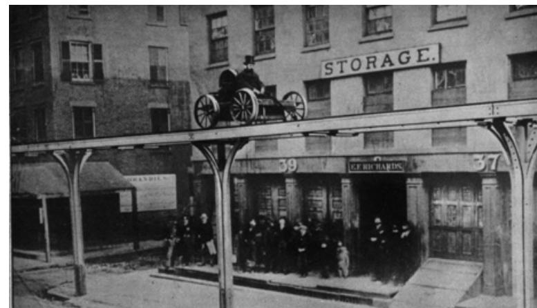
Fig 4 Charles T. Harvey Operating Car by Cable Power on First Elevated Railroad in Greenwich Street, in 1867
