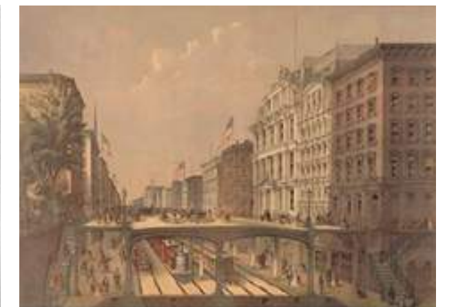
Fig. 8 The Arcade Railway
