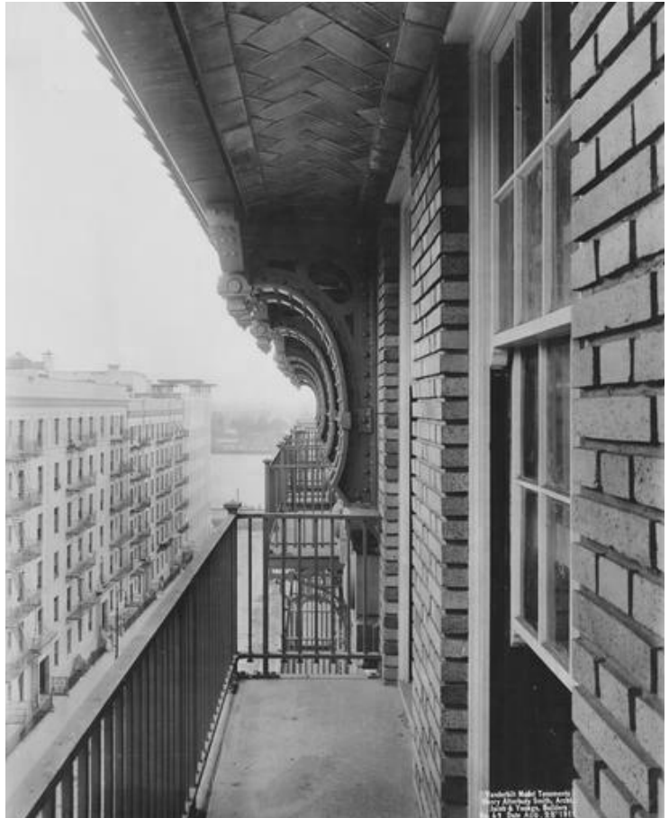
Image 08 (Right) | View of balconies at East River Homes / Shively Sanitary Tenements
