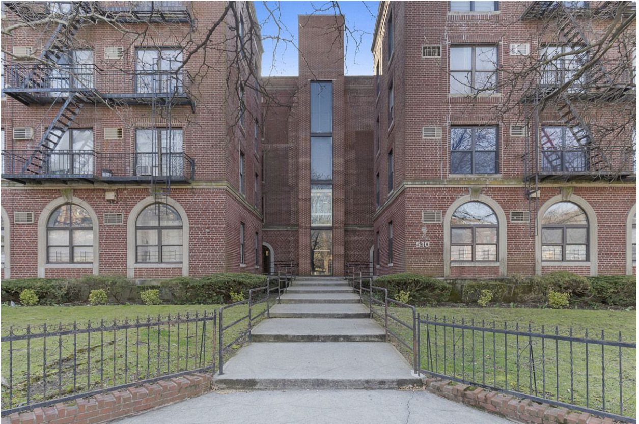
Image 12 | Entry to 510 Ocean Parkway (built 1931). An elevator addition is prominently displayed in the front yard.
