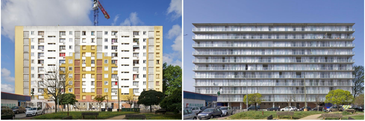
Image 10 | Before and after of the apartment block transformation. Photograph by Philippe Ruault.
