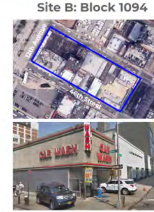
Address: 47th St and 12th Ave Current Use: Car Wash/Car Dealership Owner: Private Zoning: M2-4 (2.0 FAR)
