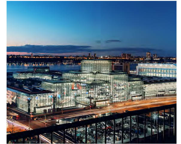
Javits Center Expansion Source: Javits Center
