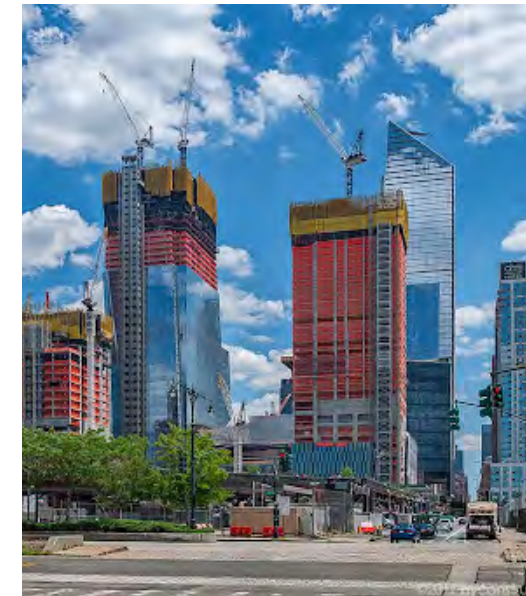
Hudson Yards Under Construction Source: Hudson Yards
