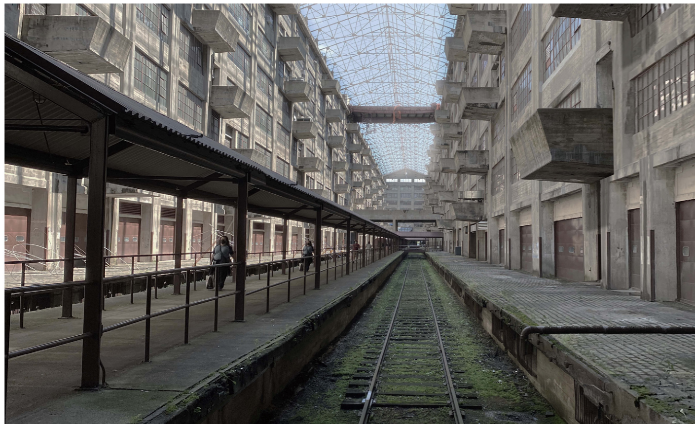
Building B atrium - existing condition
