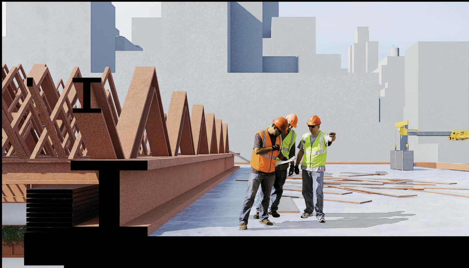
1.2. The retreat of the enclosure: For the purpose of fresh air, the workers first took off the roof enclosure.
