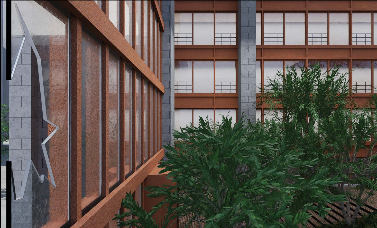
2.1. The cracking of glass: Without the maintenance, the front glass wall begins to develop dirt and stain, which cumulates and deteriorates the sealant of the glazing unit. Humidity and condensation form and ultimately the glass cracks and breaks.
