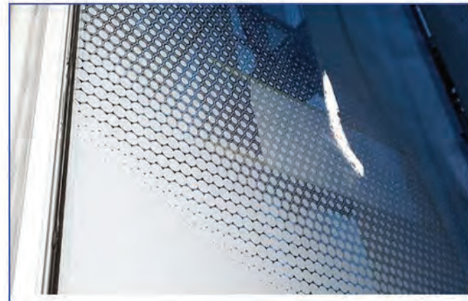
DOUBLE PANED IGU WITH CERAMIC GRADIENT FRIT
