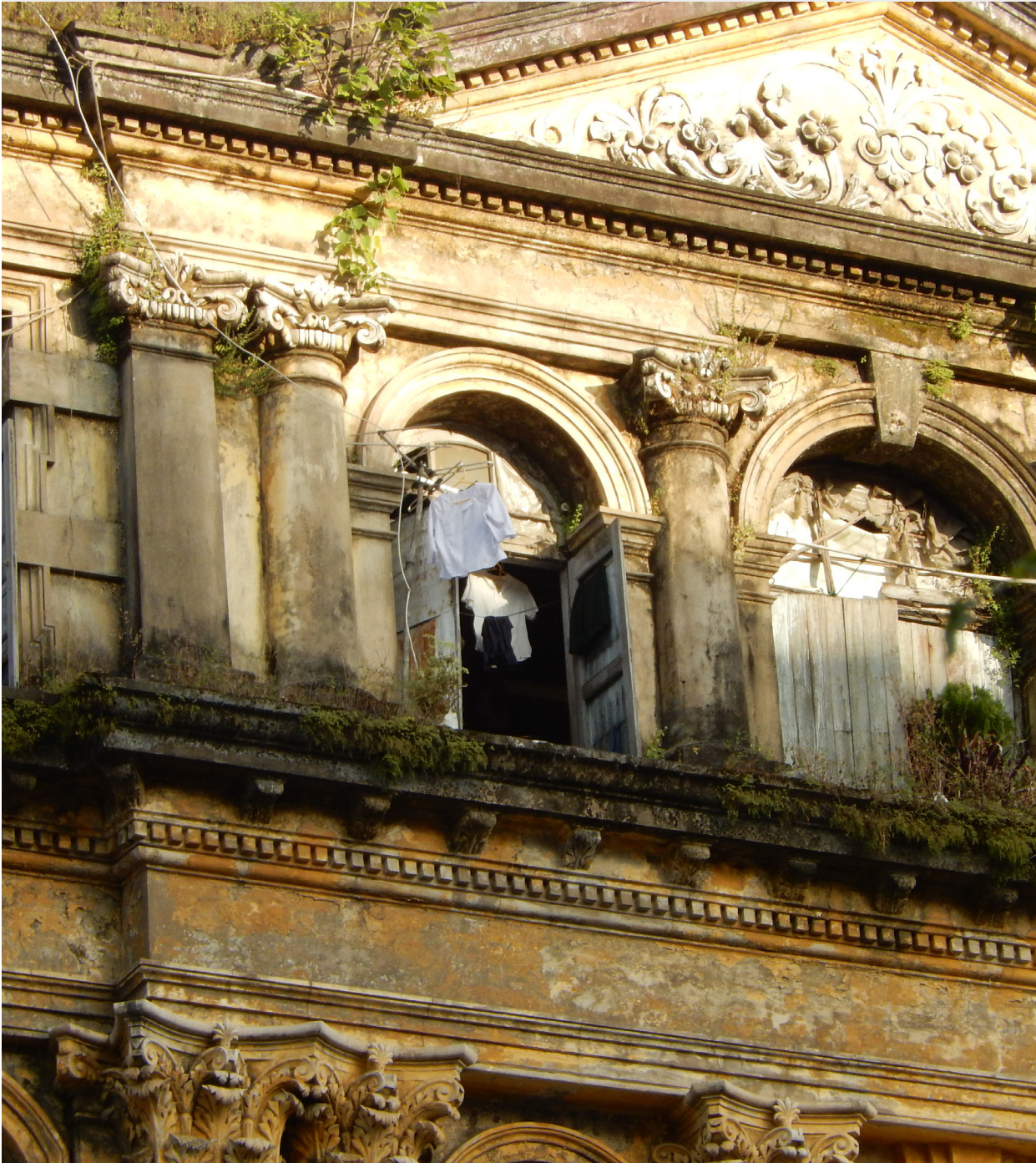
Image 43 - Vegetative growth on facades and poor building maintenance are common in Yangon's CBD
