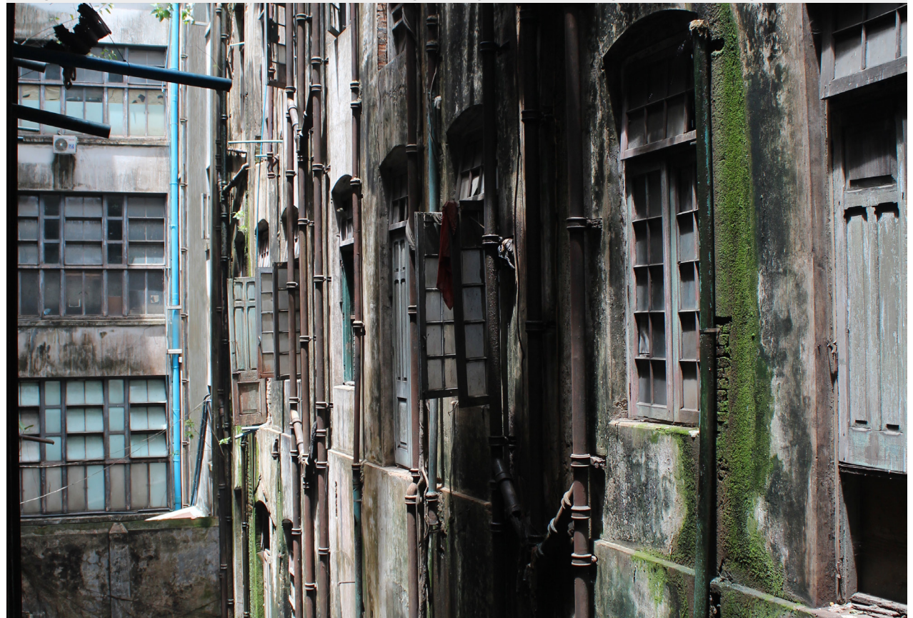
Image 42 - The interior courtyard of residential buildings in Yangon’s CBD show significant weathering
