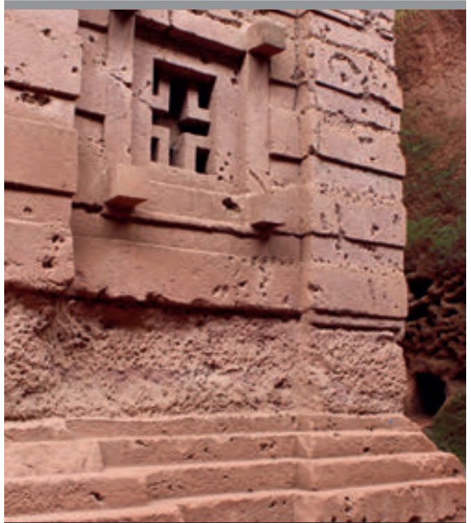
Nail marks left from early restoration on Biete Amanuel
