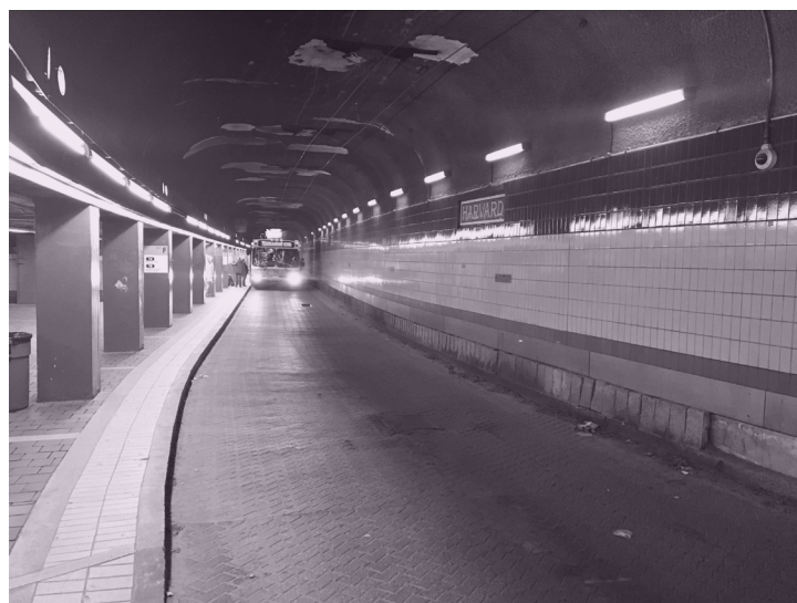
Image 1: A northbound bus operating in the Harvard Bus Tunnel Source: Author
