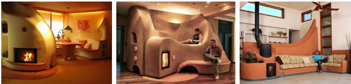
Figure 3: Earthen rocket mass heaters, an energy superefficient heating system that often includes heated benches and other interior elements. Photos: [22], [22], [23].
