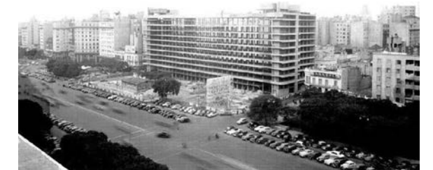
Building Under Construction
