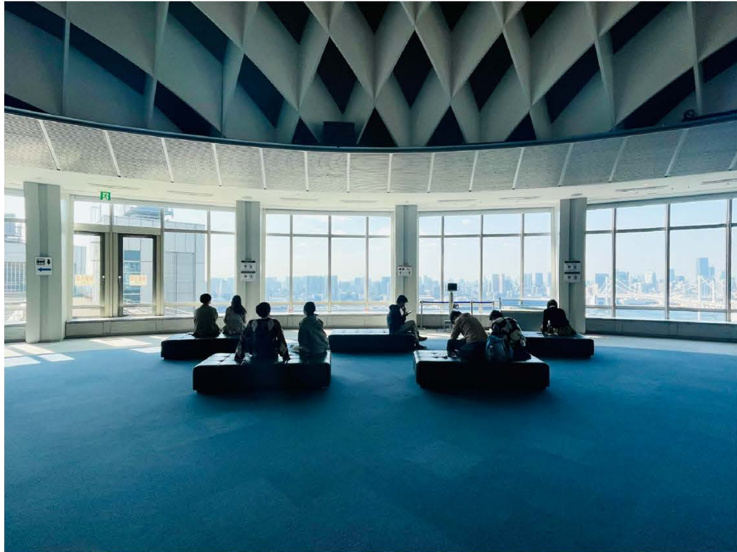
Fuji TV Headquarters - Architect Kenzo Tange
