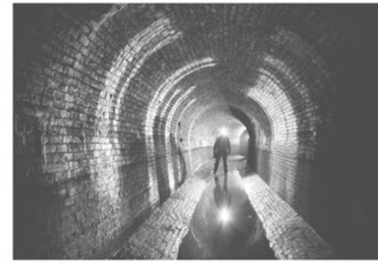
Water flows down both 85-mile-long Delaware Aqueduct and 92-mile-long Catskill Aqueduct by gravity
