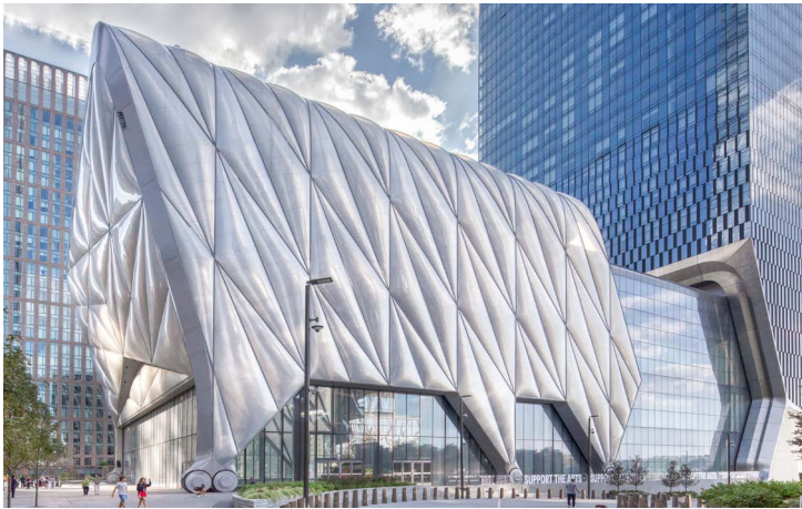
The Shed's façade from the north across Hudson Yards Public Square. (Photo: Brett Beyer.)
