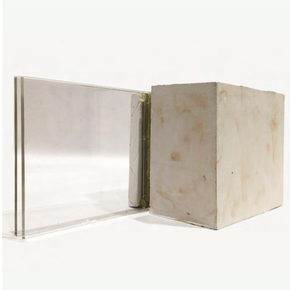
1:1 model of stone & window connection on bridged portion of through-housing units.
