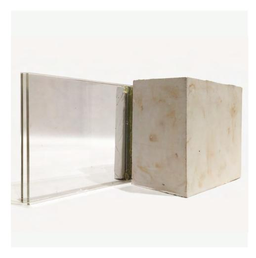
1:1 model of stone & window connection on bridged portion of though-housing units.
