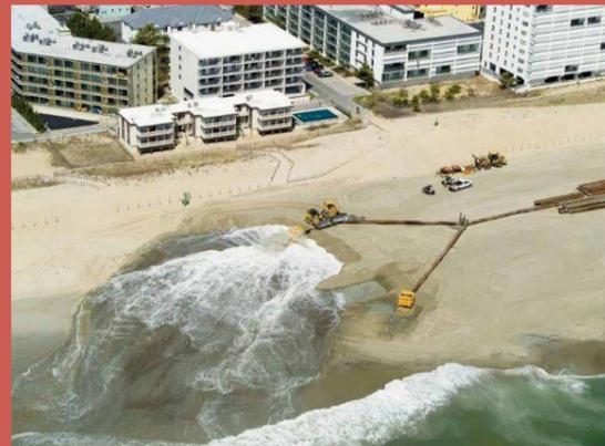
Figure 2. U.S. Army Corps of Engineers' effort to bring dredged sand to Rockaway Beach.
