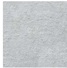
Cast-In-Place Concrete Wall
