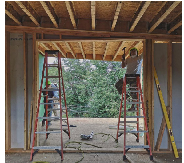
Building Project Construction Summer 2019
