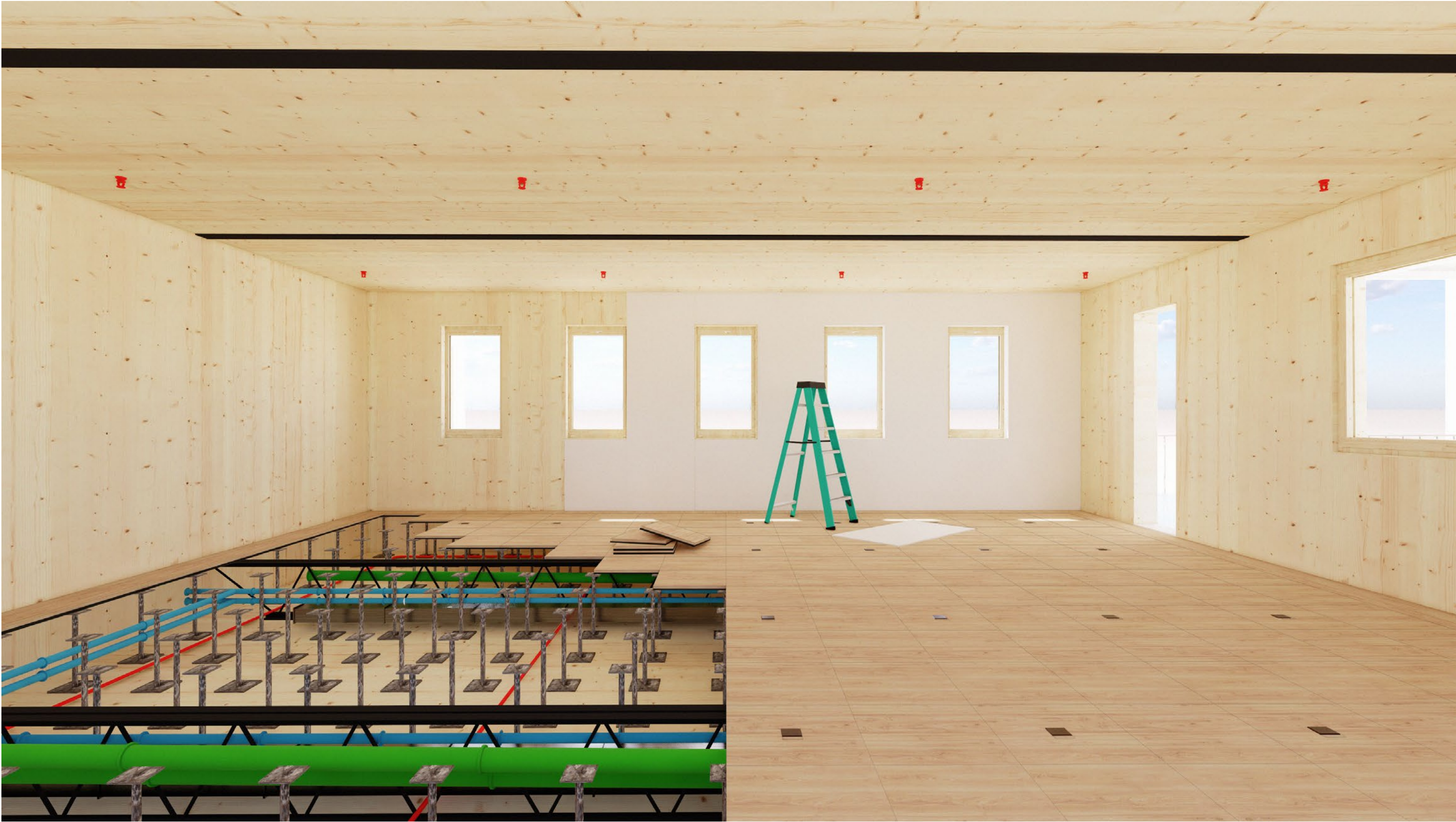
03.06 THICKEN FLOOR SYSTEMS UNDER CONSTRUCTION
