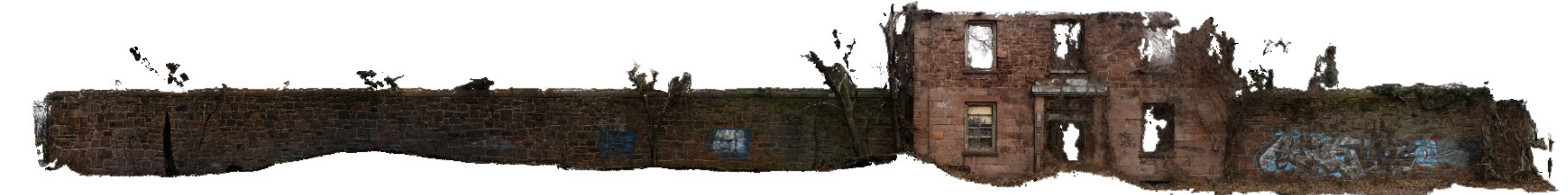
WARDEN'S RESIDENCE & PERIMETER WALL FACING NEW STREET
