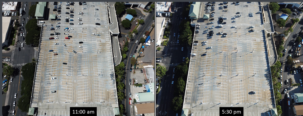
Figure 9 – Walmart/Sam’s Club parking structure at two time intervals (11:00 am and 5:30 pm)
