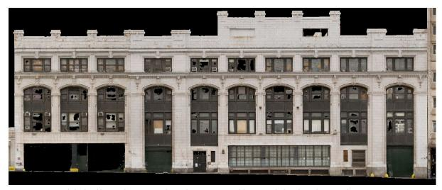
[1] In conjunction with the digital heritage documentation class, a photogrammetric model was created. The orthographic image of the facade was used to cross-reference measurements and produce a more accurate cad drawing.
