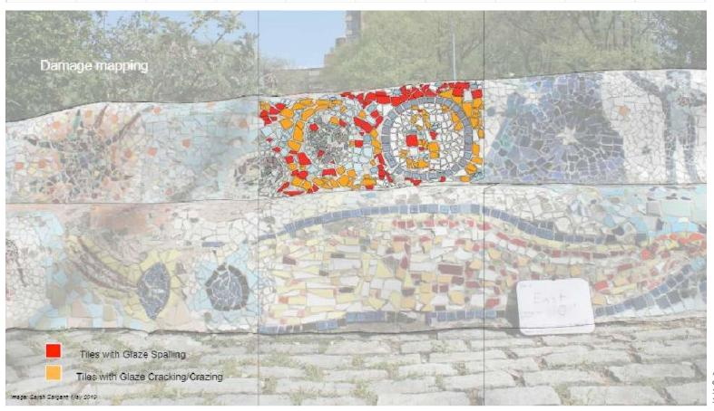
An example of a damage map created in AutoCAD Source: Prepared by Sarah Sargent
