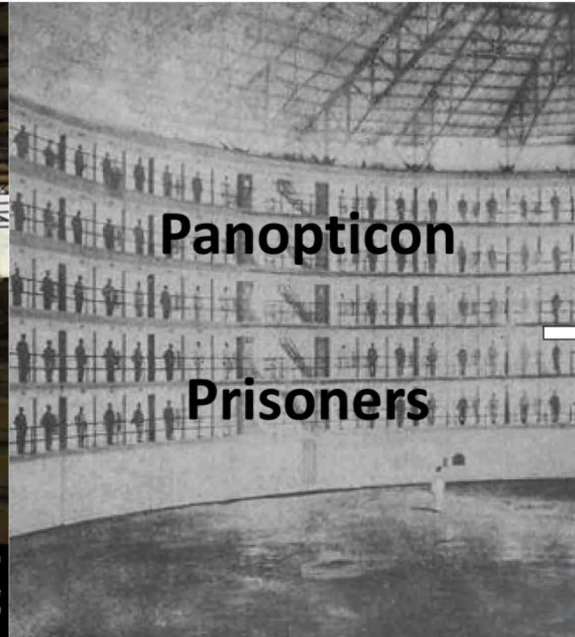
The Presidio Modelo was a "model prison" with panopticon design, built on the Isla de Pinos ("Isle of Pines"), now the Isla de la Juventud ("Isle of Youth"), in Cuba. It is located in the suburban quarter of Chacón, Nueva Gerona. The prison was built under the President-turned-dictator Gerardo Machado between 1926 and 1928. The five circular blocks, with cells constructed in tiers around central observation posts, were built with the capacity to house up to 2,500 prisoners. The panopticon design allowed the guards to watch the prisoners constantly. The prison now serves as a museum and has been declared a national monument. The old administration building now serves as a school and research center.
