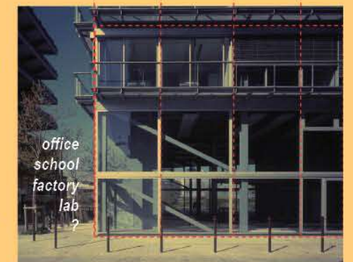
fig.4 the all-glass facade, Nantes School of Architecture, Lacaton & Vassal Architects
