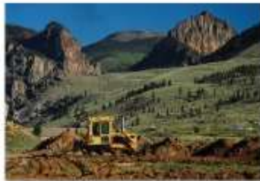
The scope of cleanup activities will depend on site size, complexity and planned reuse.
