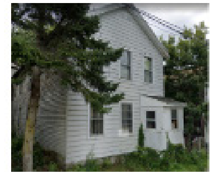
6. Demolition Project 3b1b, 2,894 sf single-family house 3b2b, 1,568 sf single-family house
