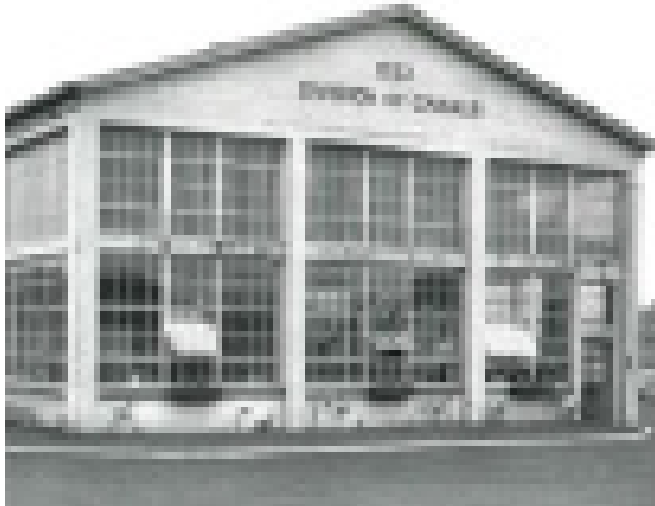
NYS Canal Corporation Building
