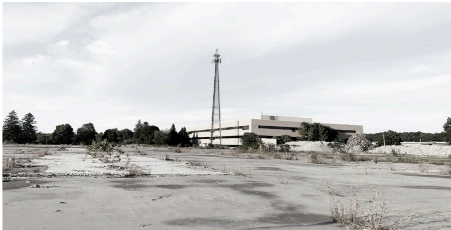
Existing IBM, photo shot on site, 10/03/2019
