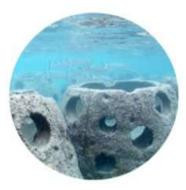
Reaf balls are structures made of concrete, slit and shells. Their porus nature that mimics reef structures provides a habitat of or aysters and other aquatic plant and fish species. The modular and cendensed versions made of recycled glass and compacted sand can be arranged and aggigated in such a way to provide a column-like support structure.
