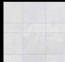
WHITE CONCRETE PANEL
