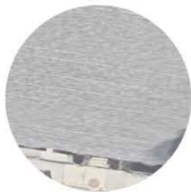
Roof Tiles Building 110
