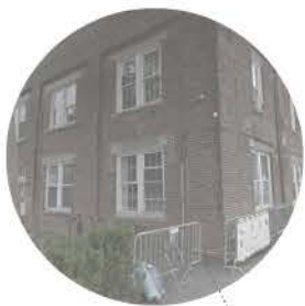
Material- Bricks Building 110
