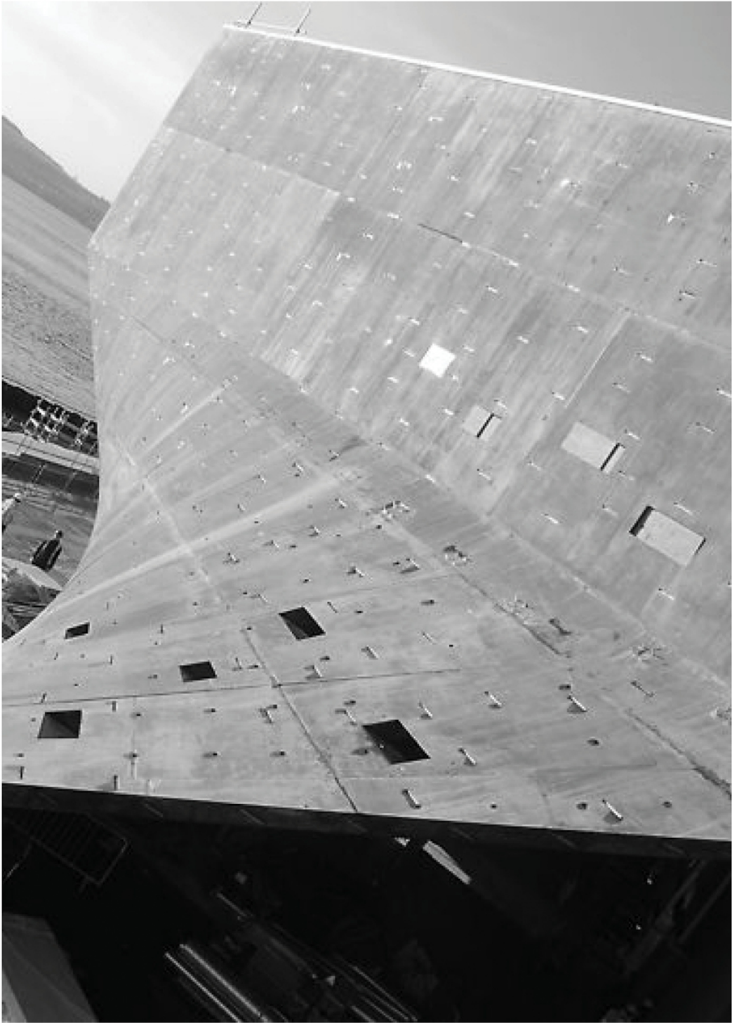
The molds for pouring concrete with three dimensional curves were made in Germany using steel plates, and transported to Dundee by ship.
