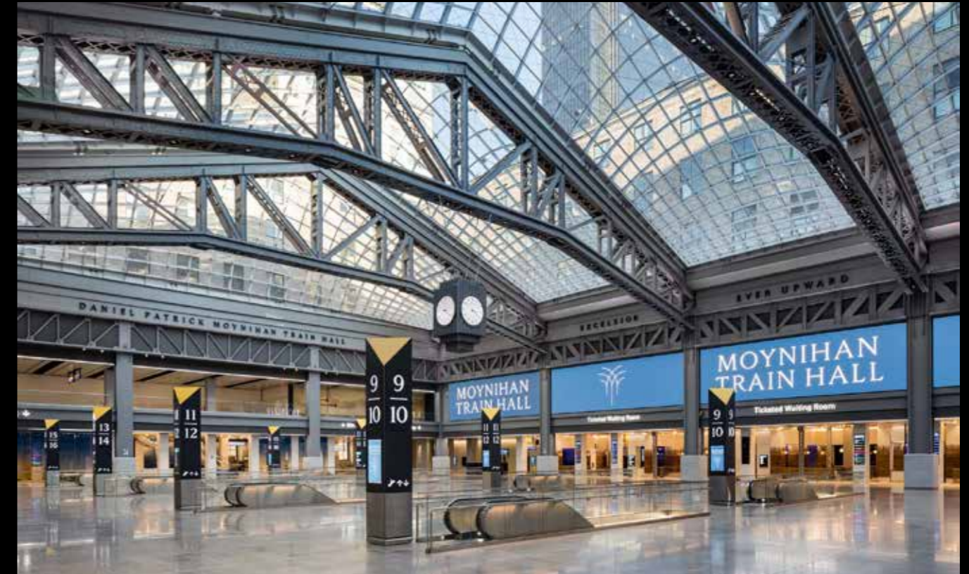
"A Grand Skylight - Sun shines through a soaring 92-foot high skylight that holds an acre of glass, 3160 insulating units—carefully housed within complex 3D steel geometrics."
