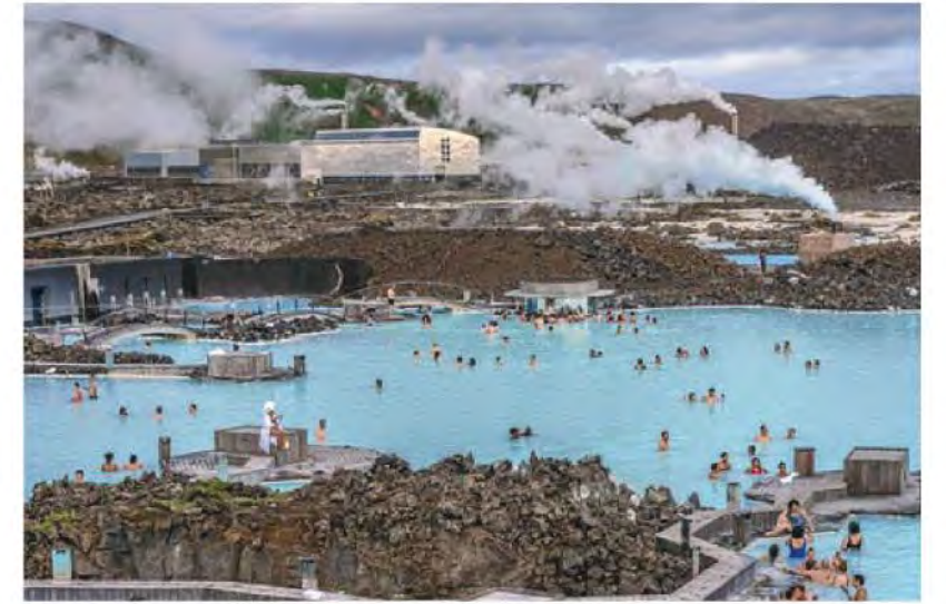
Svartsengi Geothermal Power Plant, Iceland
