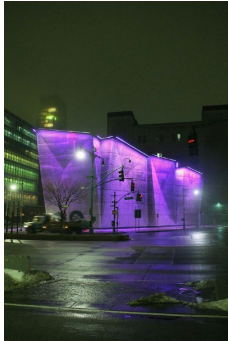
a-b. Photos of the Spring street salt shed
