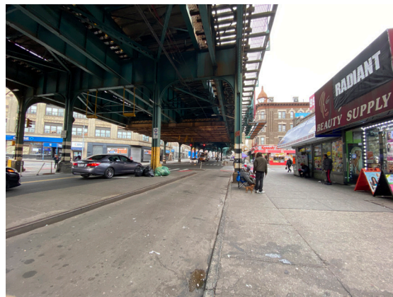
Along Jerome Avenue, one of the main commercial arteries in the area, the elevated subway lines dominate the streetscape. Around it, one-story commercial properties are abundant.
